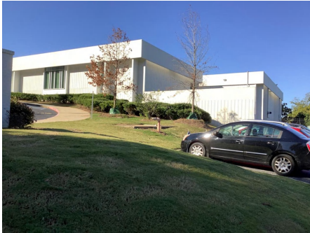
1). Northwest Elevation - Dec 26, 2019
