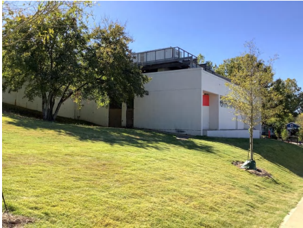
4). North Elevation - Dec 26, 2019
