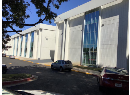
6). Southwest Elevation - Dec 26, 2019
